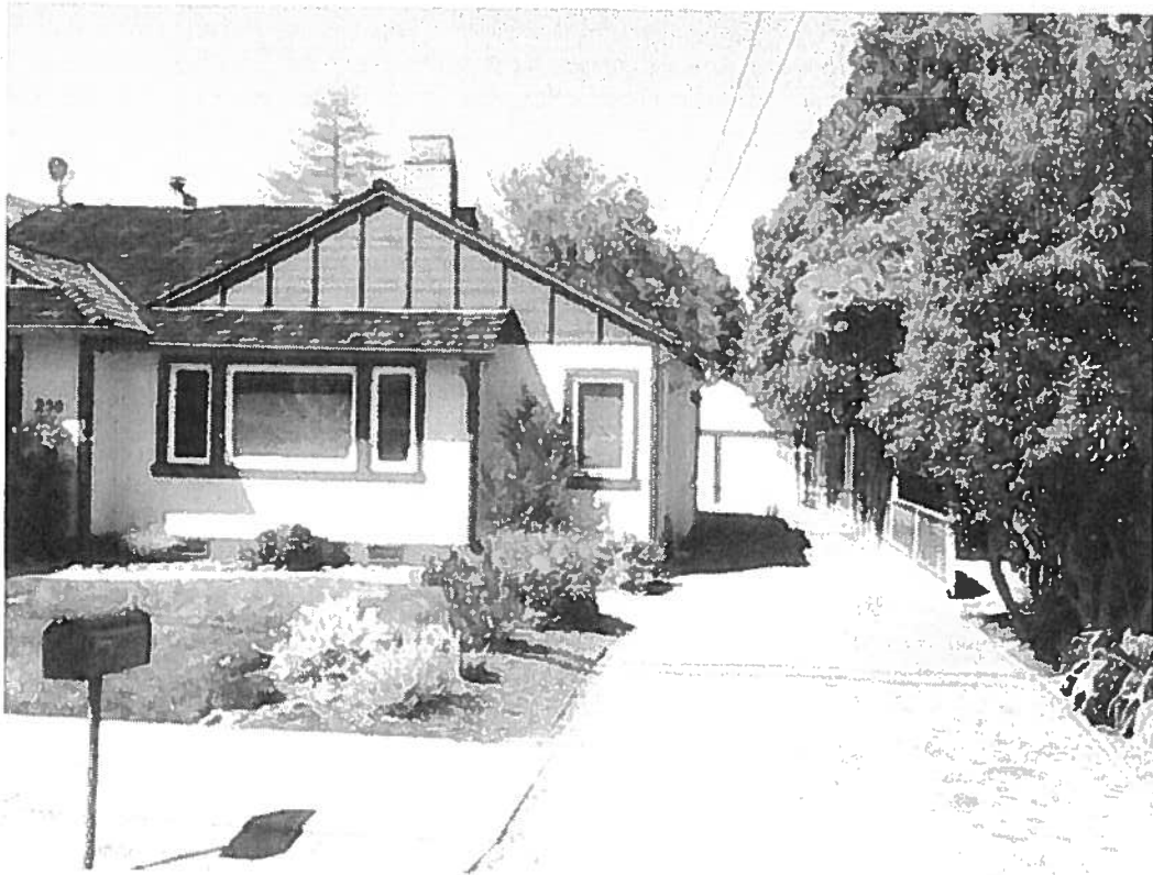
Figure 6. Photograph showing immediately adjacent property at 250 University Drive. The property under consideration and tree are located to the right. Please note the lack of any apparent damage to driveway and other structures. Please also note the significant overgrowth of the property boundary via additional non-heritage plants and trees due to apparent negligence.
