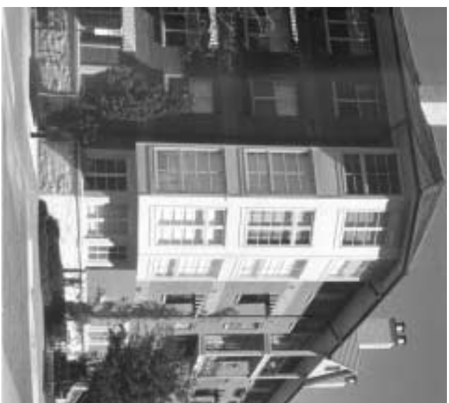
A stone base, brick middle, and roof overhang delineate the three “layers” of this new building.
