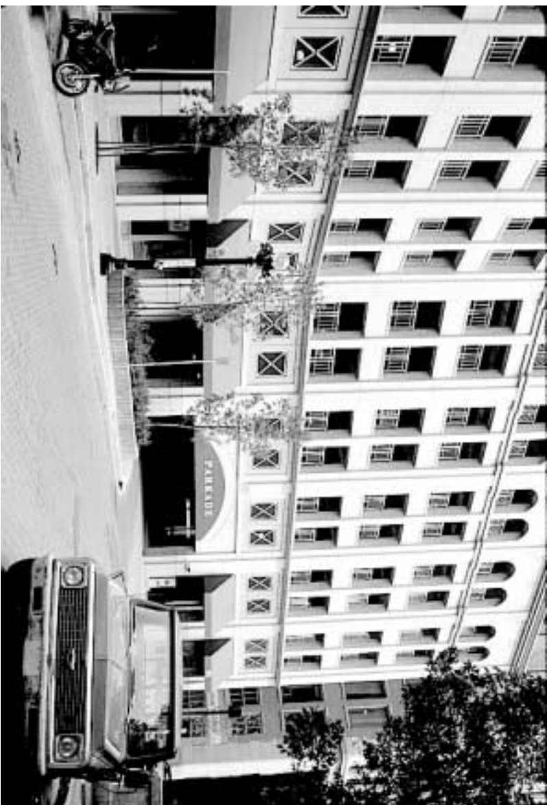
This structure has the appearance of a typical commercial building rather than a parking ramp. The punched openings at the parking levels relate to the window proportions of surrounding buildings.
